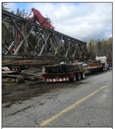
Moving the bridge required lifting it with an excavator and a loader, while the float truck positioned itself underneath.
